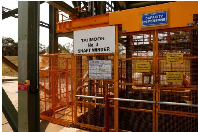
Photograph 1: Tahmoor No.3 shaft winder. Photograph by Resources Regulator
