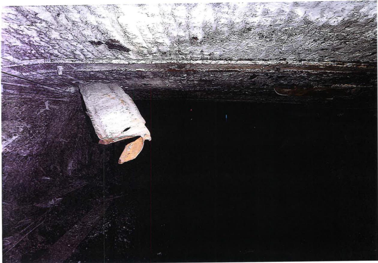
Photograph of the damaged W Strap hanging down into the roadway. *Photograph taken by the mine.*
